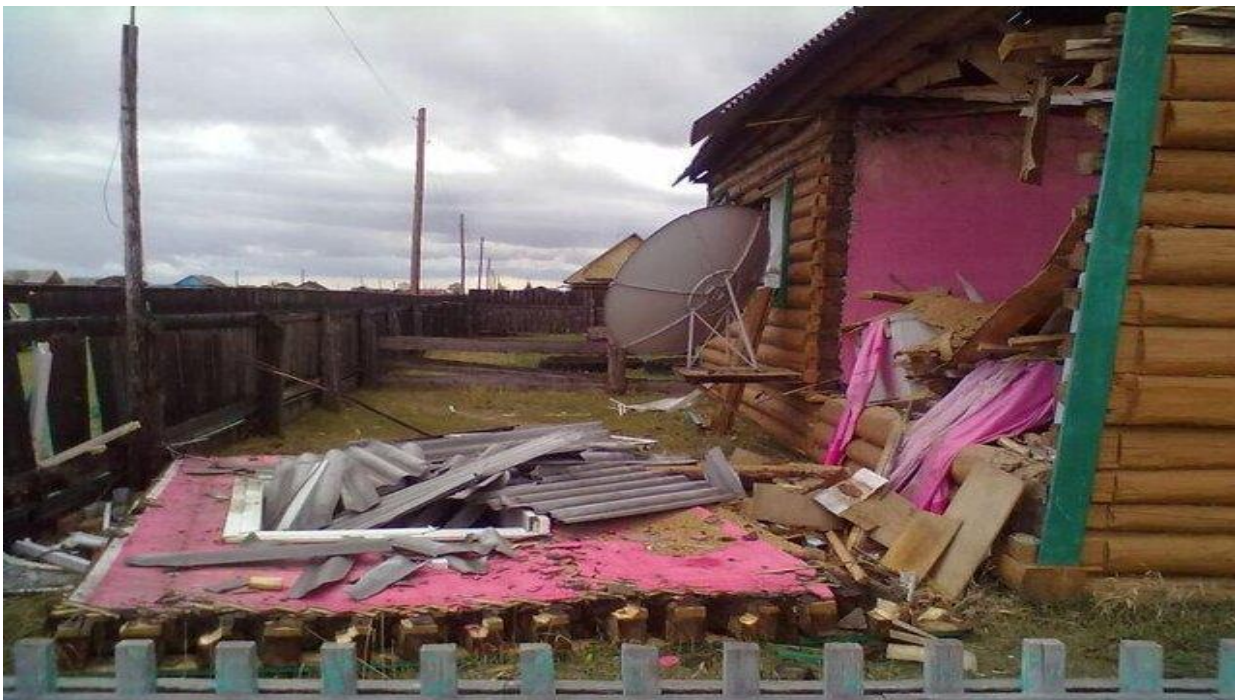
Figure 1. The house wall thrown out by the explosion. Adapted from “Sources and components of ball lightning theory” A I Nikitin et al 2018 J. Phys.: Conf. Ser. 996 012011.
