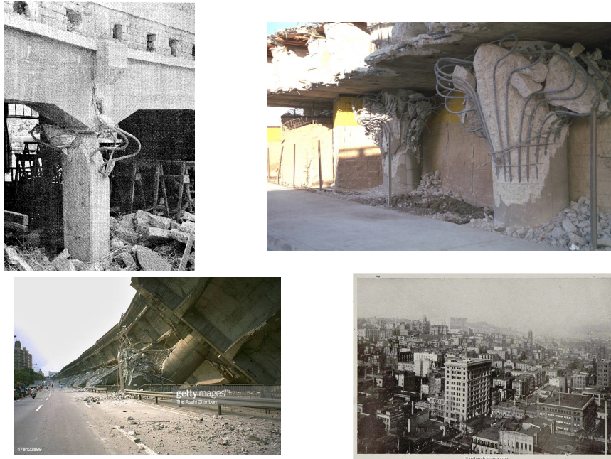
FIGURE 9. Characteristic building damages from a suspected nuclear earthquake in Tangshan 1976 and two other nuclear earthquakes in Northridge 1994 and in Hanshin 1995. Relatively light building damages from a natural M_w 7.9 earthquake in San Francisco 1906 at only a hypocentral distance of 15.5 km and triggered by the rupture of the giant San Andreas Fault.
