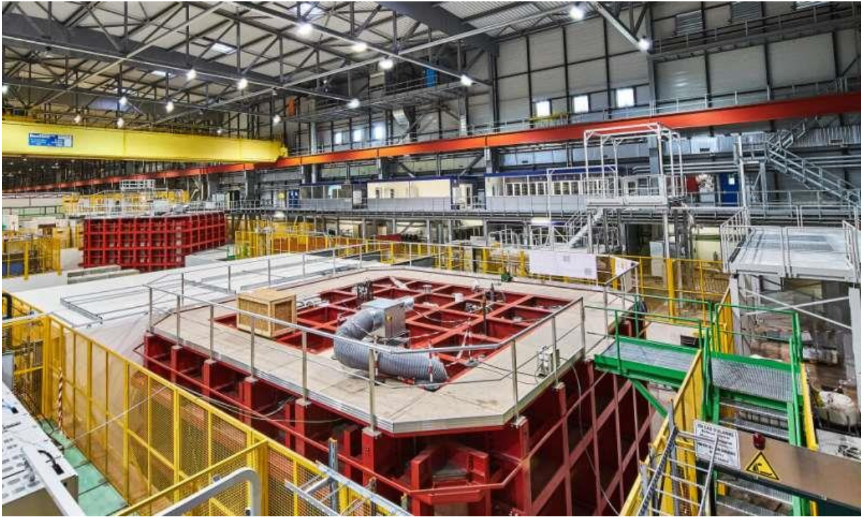
The outer structures (red) for two prototype DUNE detectors that are currently being evaluated at CERN. (Image: CERN)
