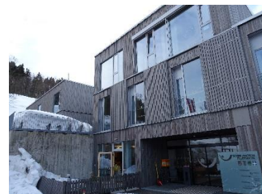
Fig. 6. Entrance to Social Center Pillerseetal with kindergarten to the left.
