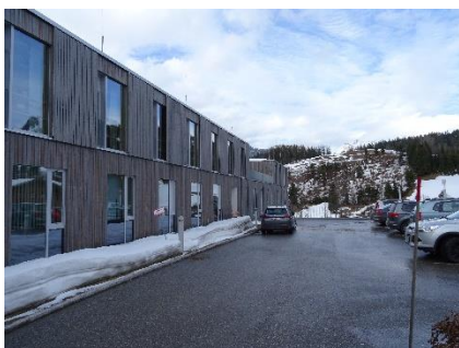
Fig. 8. Part of Social Center Pillerseetal with two floors of stacked CLT module rooms.
