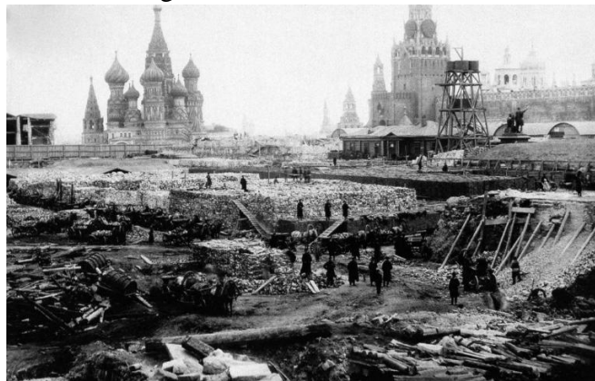
Fig. 6. Excavations on Red Square, Moscow, at the end of the 19th century. 150 m above sea level.
