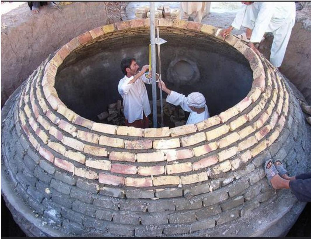
*Figure 68. A dome under construction*
