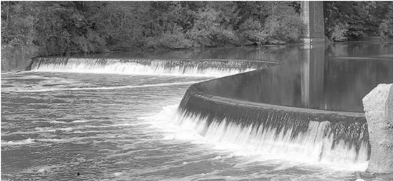
**Figure 8. Curves in dams are made to increase their strength like with arches.**
