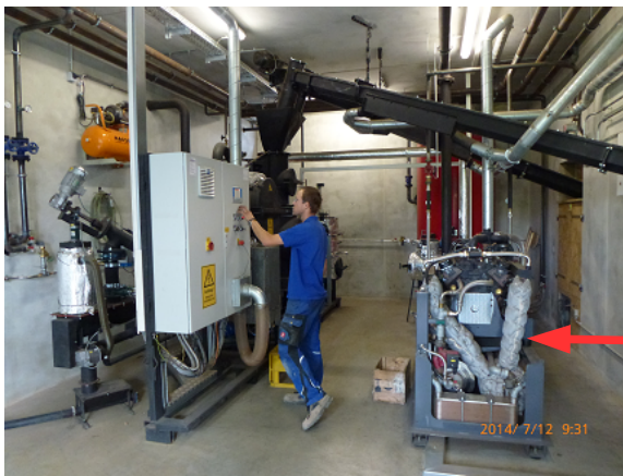
Fig. 5. Spanner Re 2 wood gas cogenerator installed by Josef Strobl Heizung Solar in Giglberg and Velden/Vils/Lower Bavaria/Germany. Left: pyrolysis unit in left image half. Gas engine and generator on right half. Right: enlarged image of Gas engine and generator.
