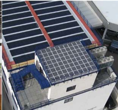
Stair and lift roof
