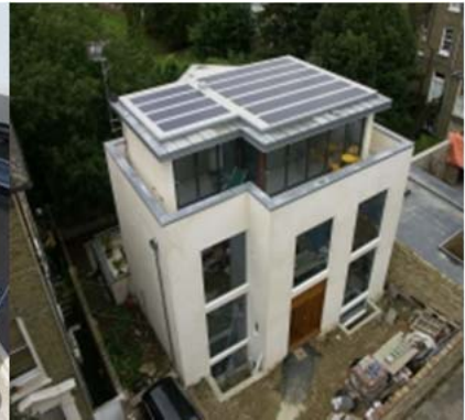
'Eaton Rise' Single family house
