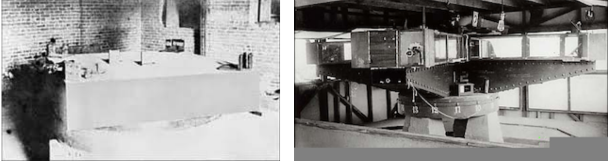
Figure 1: Left: Michelson-Morley interferometer experiment of 1887. Right: Miller 1925/26 interferometer experiment. Examples of detected fringe shifts on rotation shown in Fig.4, after extracting the temperature and non-orthogonal mirror effects.
