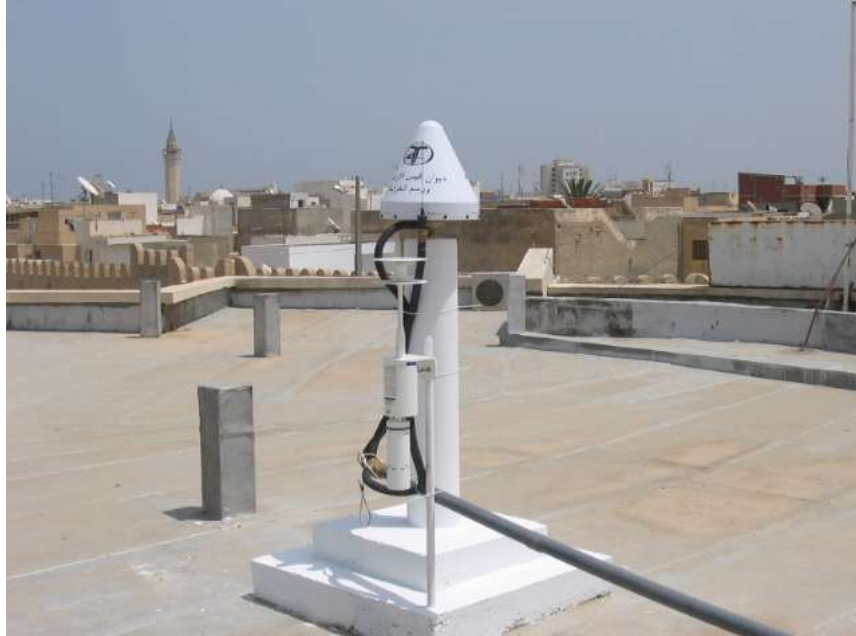
Figure 7 : la Station GPS Permanente de Monastir
