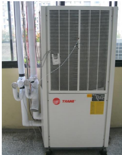
Figure 1. Air-cooled chiller
