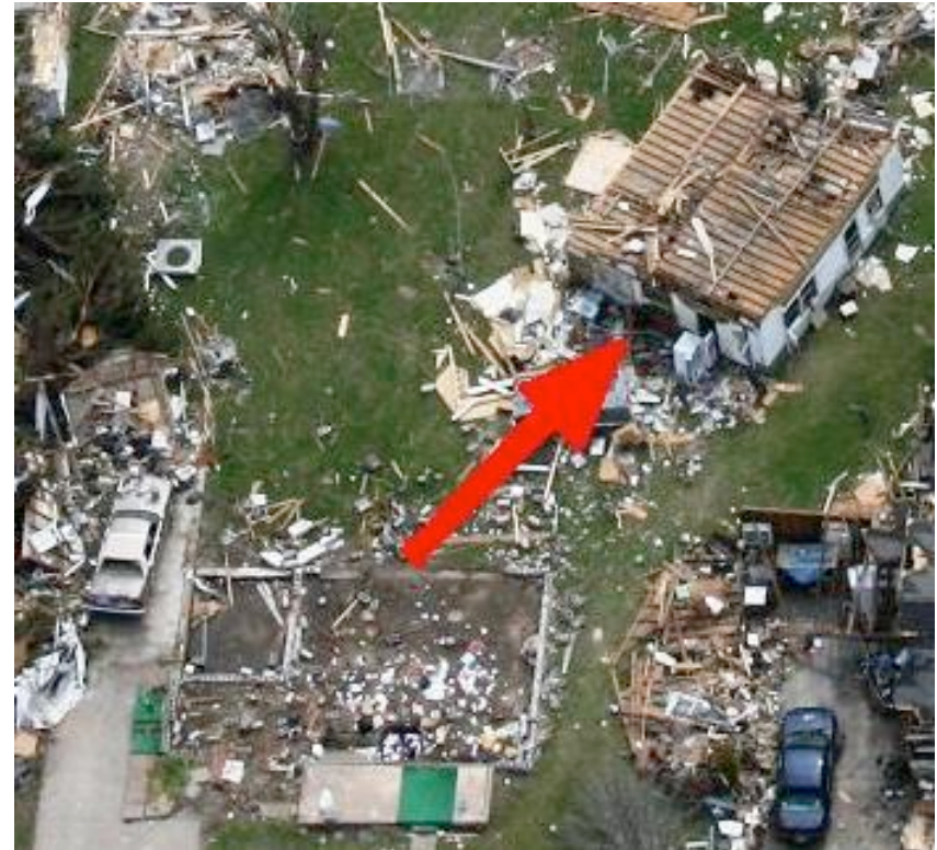
Figure 117. House relocated by the EF5 tornado in Greensburg, KS, 2007-05-04, courtesy Tim Marshall .
