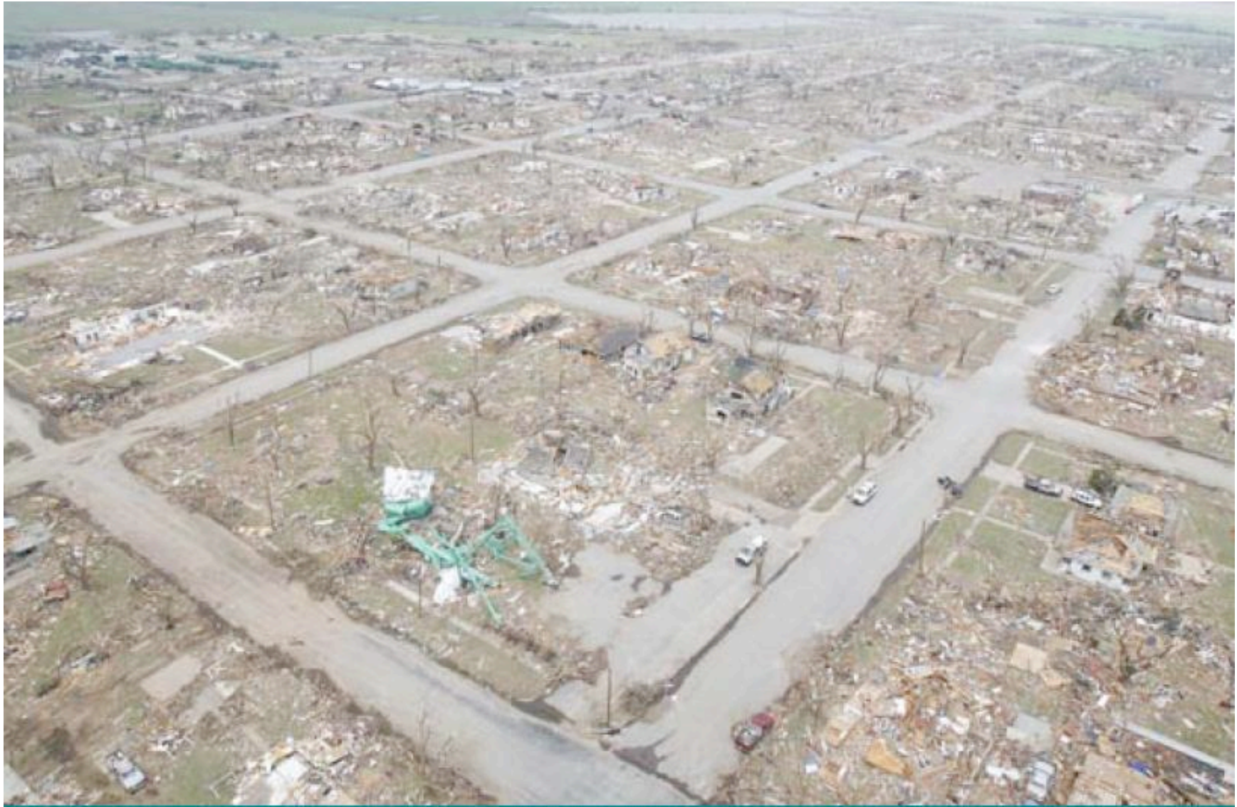
Figure 6. Damage from an EF5 tornado in Greensburg, KS, 2007-05-04, courtesy FEMA .
